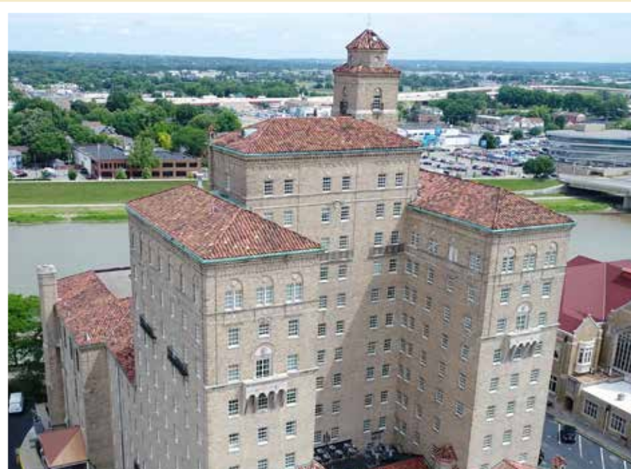
6 The Dayton YMCA building opened in 1928 with 13 stories, 13 classrooms, three gyms, a pool, library, auditorium, 245 residence rooms and more.
