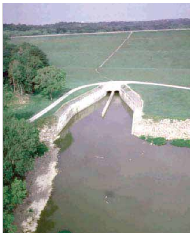
Englewood Dam is one of MCD's five flood protection dams.
