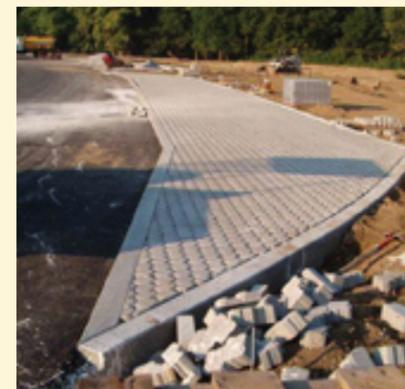
Pervious brick pavers are installed to allow runoff to seep into the ground.
