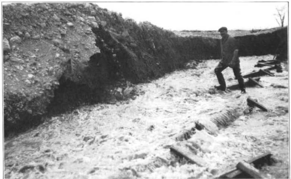
FIG. 187—SLUICE DITCH UNDERMINING AND EXCAVATING THE BORROW PIT FLOOR. JUNE, 1920
