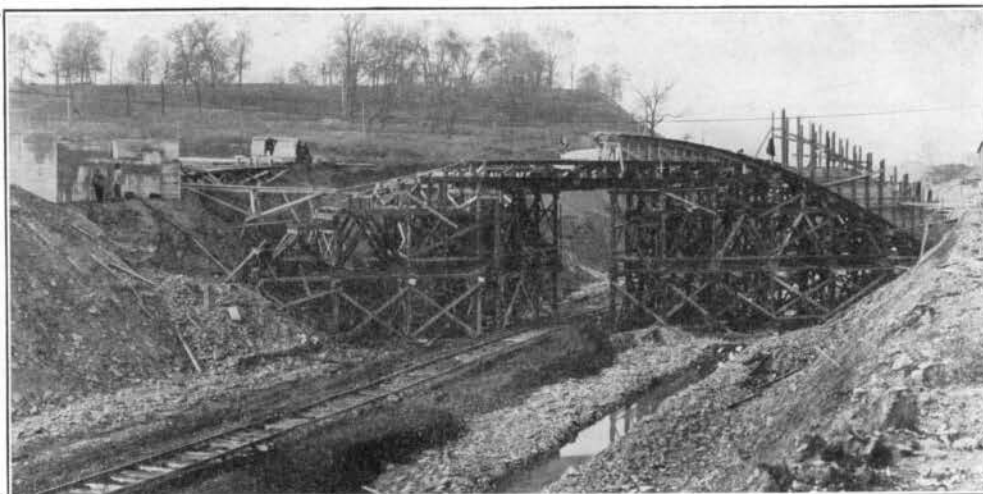
FIG. 178—FALSEWORK FOR HUFFMAN THREE-HINGED ARCH BRIDGE. OCT. 22, 1919.
