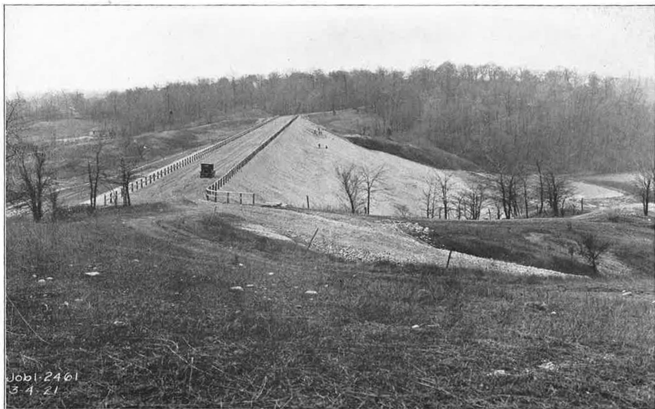
FIG. 289—HIGHWAY CROSSING TWIN CREEK VALLEY ON CREST OF GERMANTOWN DAM, MARCH 4, 1921.
