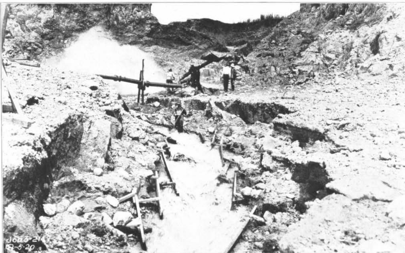
FIG. 184—MONITOR TEARING DOWN LOCKINGTON PIT FACE. AUG. 5, 1920. SEE PAGE 20
