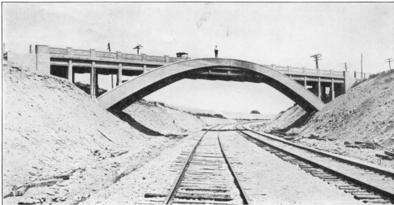
FIG. 177—THREE-HINGED ARCH SKEW BRIDGE AT HUFFMAN. JUNE 26, 1920.
