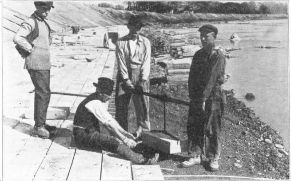
FIG. 224—LAYING FLEXIBLE CONCRETE REVETMENT, OCT. 30, 1920
