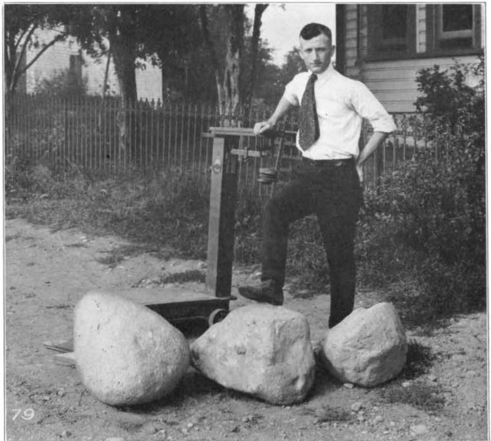
FIG. 193—LARGE STONES WHICH HAVE COME DOWN THE LOCKINGTON SLUICE DITCHES. TAKEN AUGUST 23, 1920
