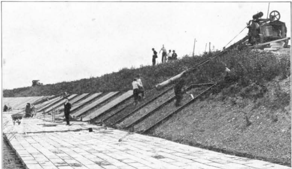
FIG. 225—CASTING THE CONCRETE REVETMENT SLABS, JUNE 2, 1920
