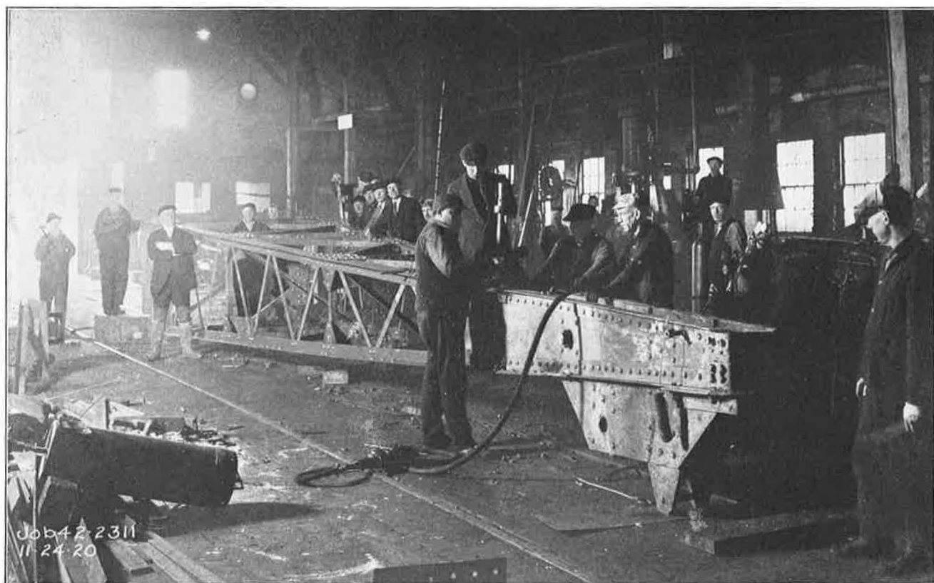
FIG. 248—REPAIRING DRAGLINE EXCAVATOR BOOM IN CONSERVANCY SHOP, NOV. 24, 1920.
