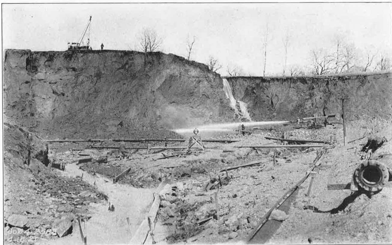
FIG. 318.—HYDRAULIC GIANTS EXCAVATING MATERIAL IN THE BORROW PIT AT TAYLORSVILLE, APRIL 18, 1921
