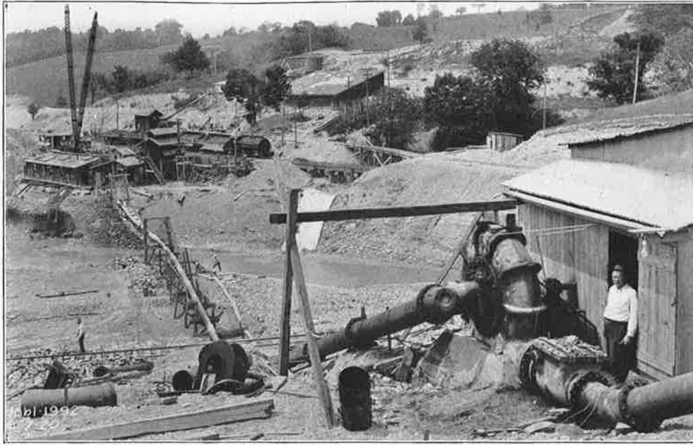
FIG. 298—WHITE IRON BOOSTER PUMP, GERMANTOWN DAM, JUNE 1, 1920
