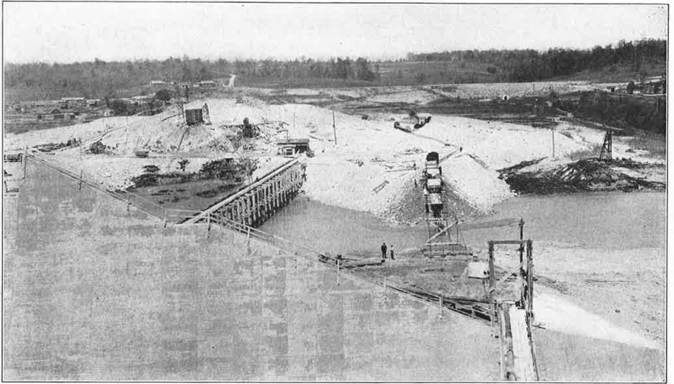
FIG. 319.—CLOSING THE OLD RIVER CHANNEL AT TAYLORSVILLE DAM, MAY 5, 1921.
