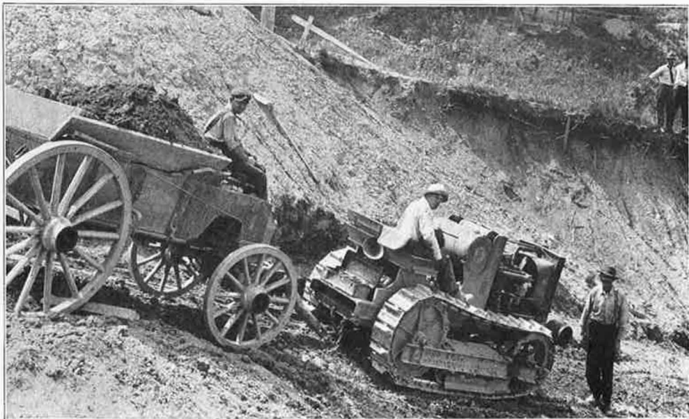
FIG. 328.—HANDLING LOADED WAGONS ON A STEEP SLOPE AT TAYLORSVILLE, JUNE 1, 1921.
