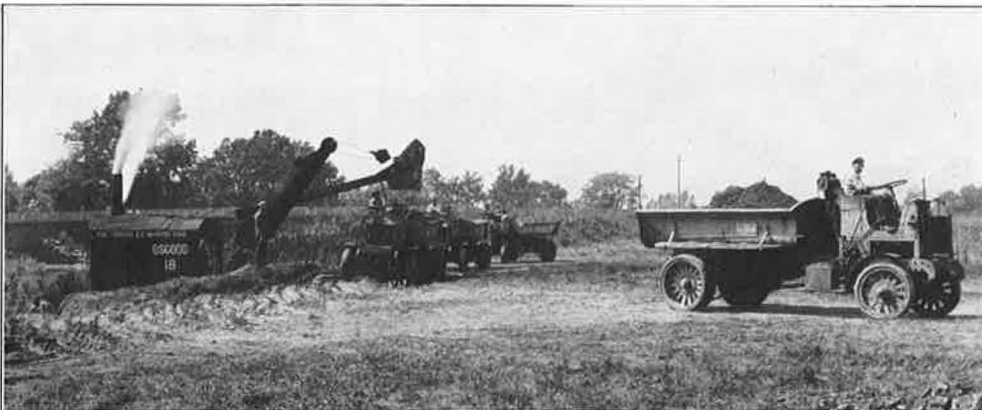
FIG. 315—TRANSPORTING EARTH IN SEVEN-TON TRUCKS, SEPT. 7, 1920
