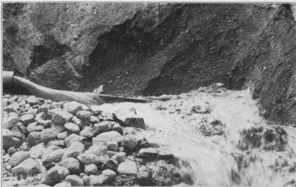
FIG. 185—SLUICING LOOSE GRAVEL AT LOCKINGTON. AUGUST 5, 1920
