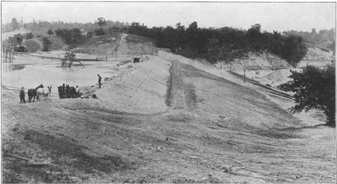
FIG. 170—LOOKING NORTHERLY ACROSS THE GERMANTOWN DAM. JUNE 7, 1920.
