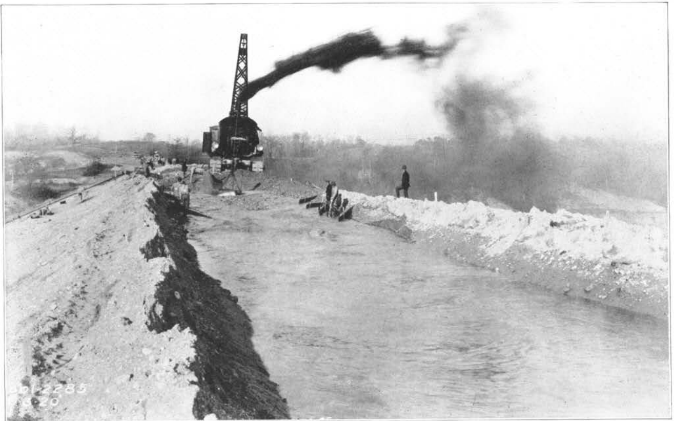
FIG. 228—TOPPING OUT THE GERMANTOWN DAM, NOVEMBER 3, 1920
