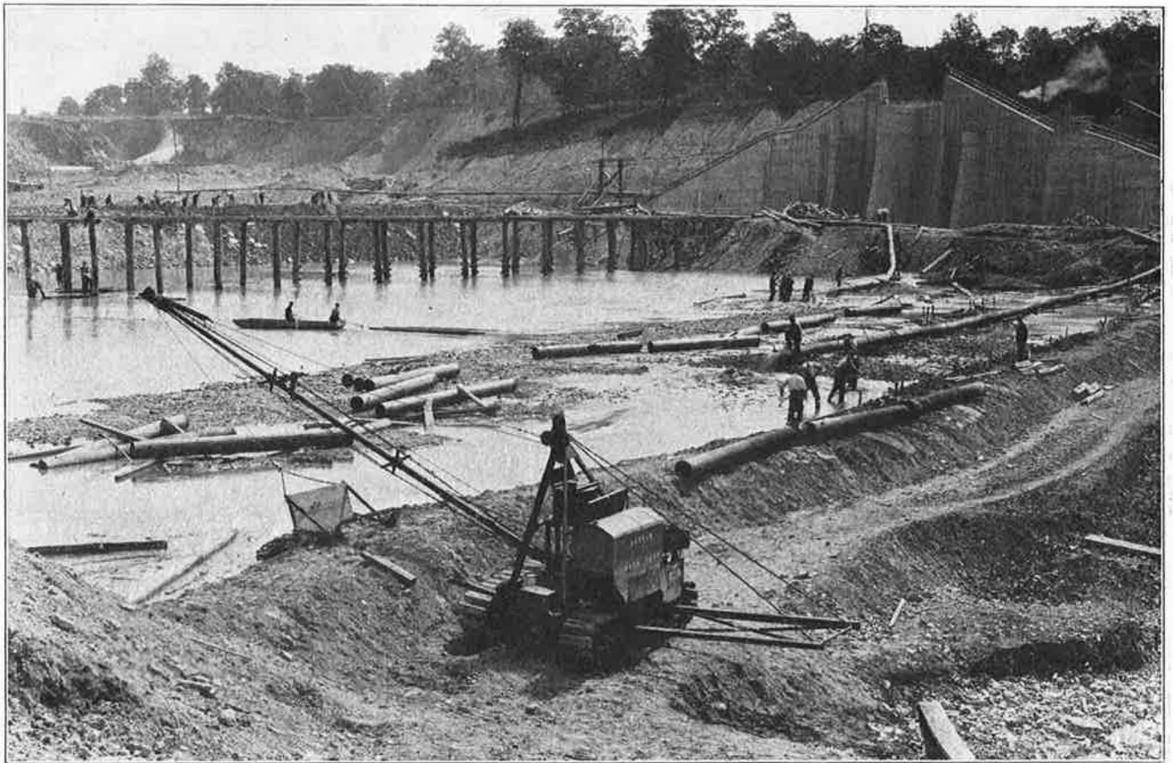
FIG. 320.—SLUICING MATERIAL INTO OLD RIVER CHANNEL AT TAYLORSVILLE DAM, JUNE 1, 1921
