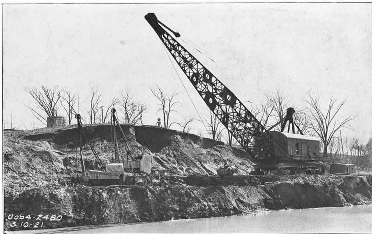
FIG. 304—ROCK EXCAVATION BELOW OUTLET WORKS, TAYLORSVILLE DAM, MARCH 10, 1921
