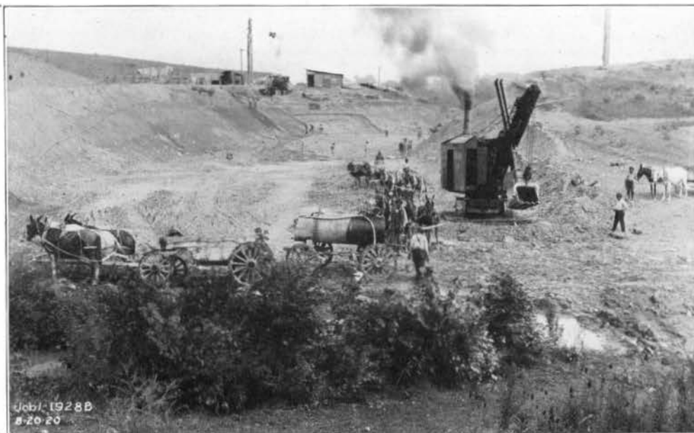
FIG. 238—EXCAVATING FOR THE GERMANTOWN SPILLWAY, AUGUST 20, 1920
