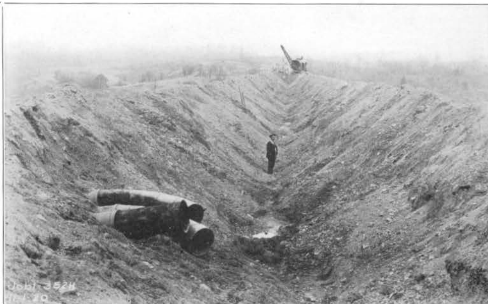
FIG. 236—RESULT OF THIRD STAGE OF TOPPING OUT GERMANTOWN DAM. NOVEMBER 3, 1920
