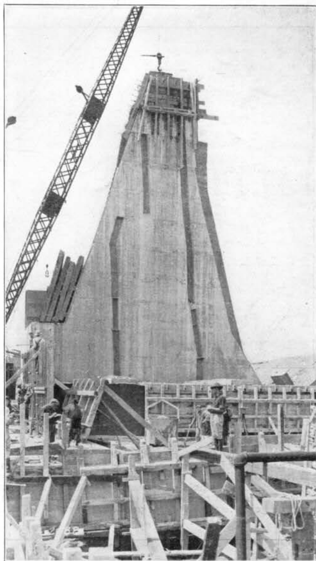
FIG. 183—WEST WALL OF TAYLORSVILLE CONDUIT OUTLET, JULY 20, 1920.
