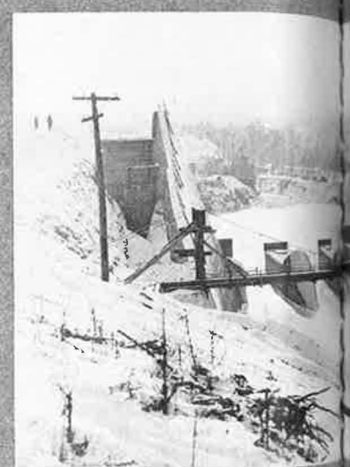
FIG. 252—PROGRESS ON THE CONSTRUCTION
