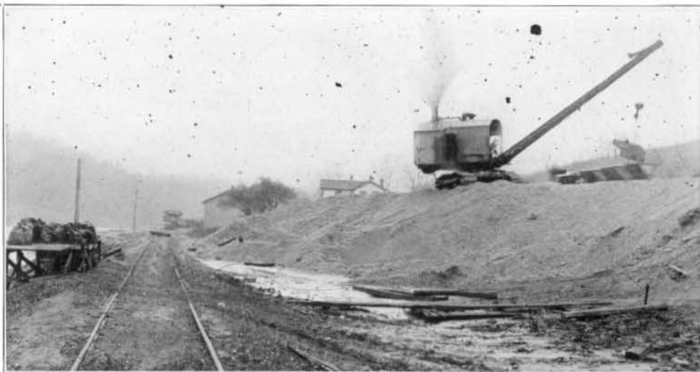
FIG. 233—LOADING CARS WITH CONCRETE "AGGREGATE," NOVEMBER 24, 1920.
