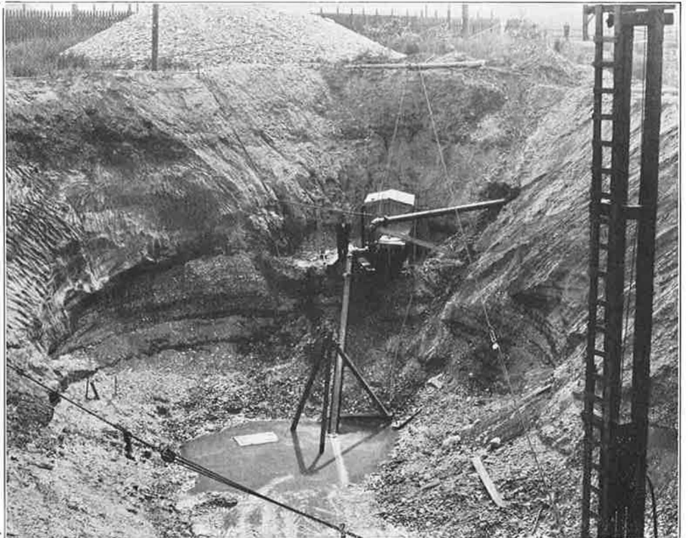
FIG. 264—PUMP "UNWATERING" ABUTMENT EXCAVATION, BLACK STREET BRIDGE, JUNE 10, 1920
