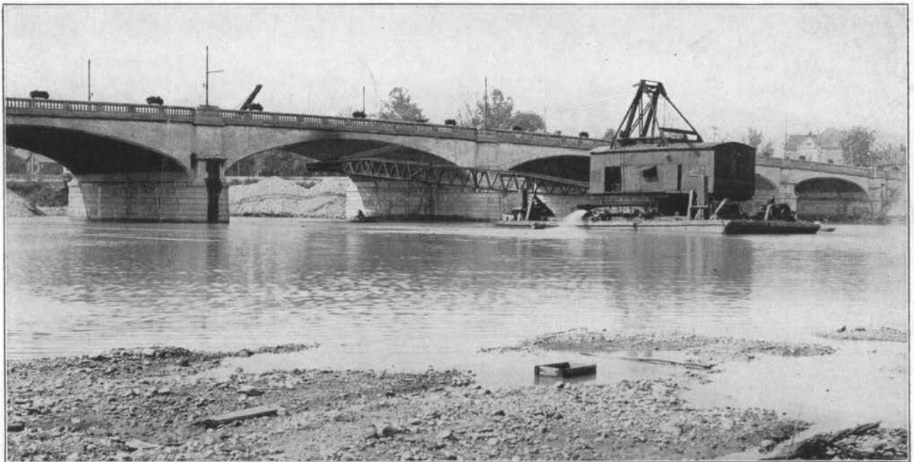
FIG. 196—EXCAVATING UNDER THE THIRD STREET BRIDGE. JULY 23, 1920
