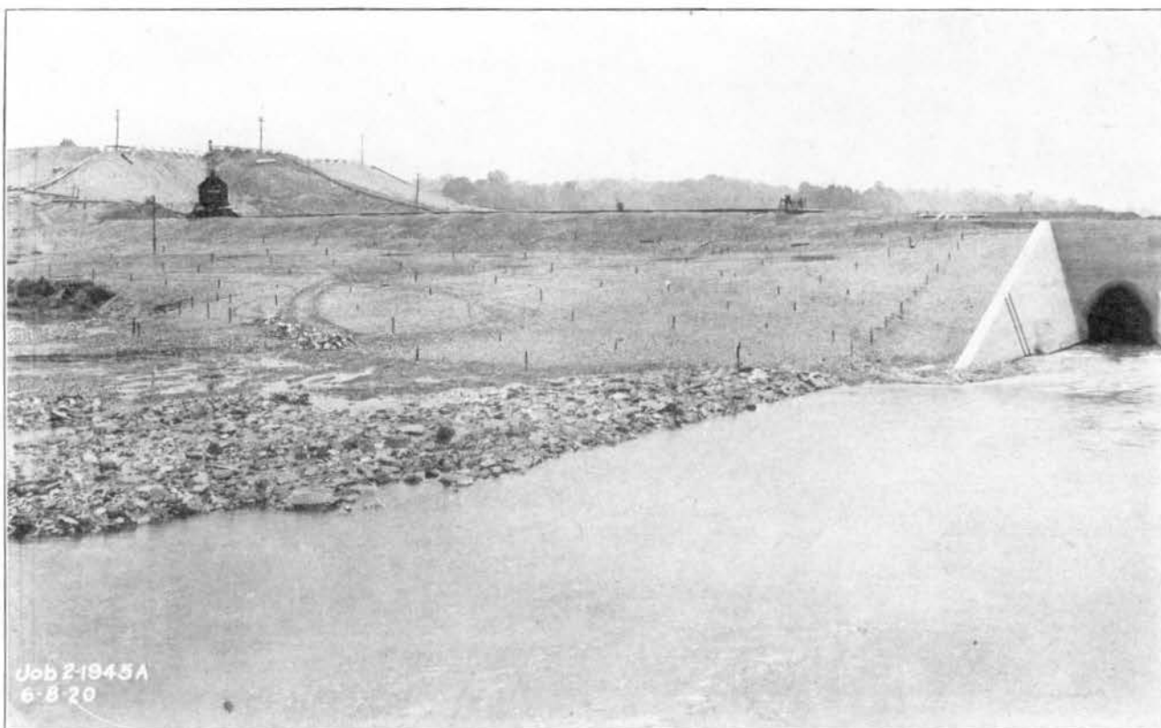
FIG. 215—RIVER SECTION, ENGLEWOOD DAM EMBANKMENT, JUNE 8, 1920
