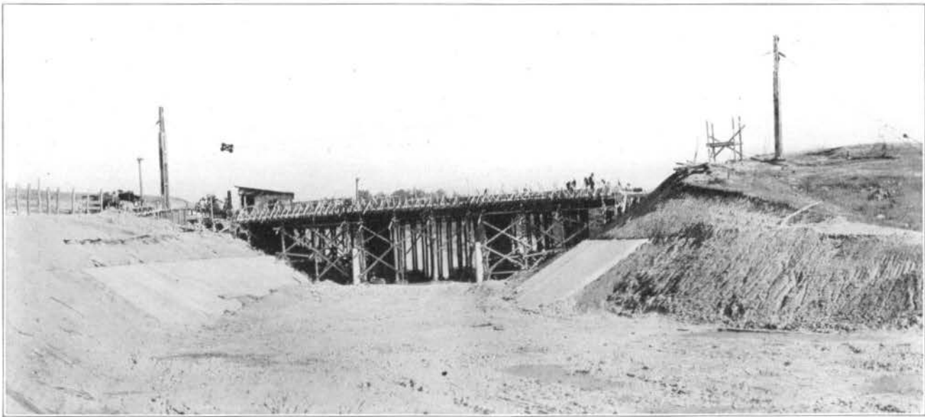
FIG. 242—BUILDING THE GERMANTOWN SPILLWAY BRIDGE, OCTOBER 13, 1920
