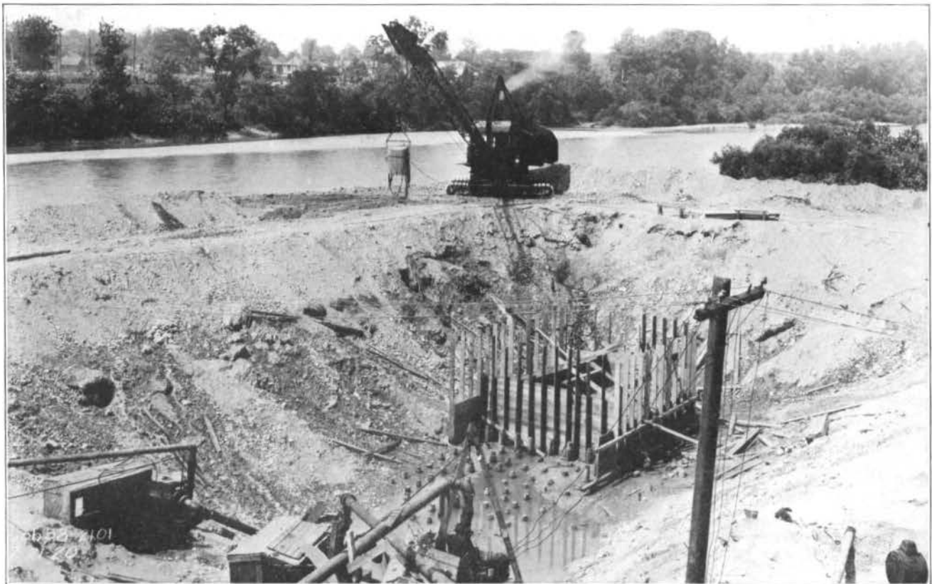
FIG. 176—OPEN EXCAVATION FOR PIER NO. 3, BLACK STREET BRIDGE, HAMILTON. JULY 21, 1920. (See the descriptive article on this page.)
