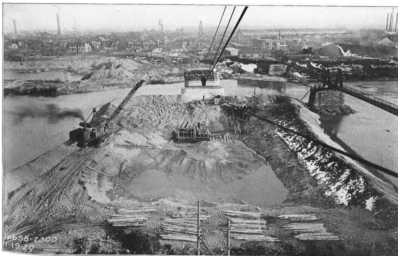
FIG. 259—EXCAVATION FOR PIERS 5 AND 6, BLACK STREET BRIDGE, NOV. 19, 1920.
