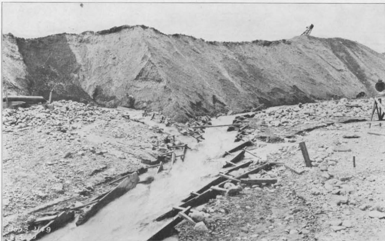
FIG. 186—GRAVEL PILE BEING SLUICED DOWN BY LOW PRESSURE WATER, AND ALSO BY A SLUICE DITCH. AUGUST 5, 1920
