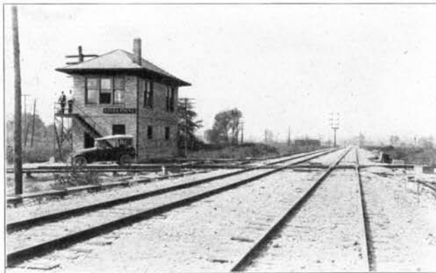
FIG. 207—INTERLOCKING PLANT AT TATES POINT. SEPT. 20, 1920.
