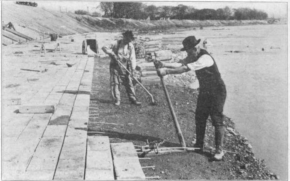
FIG. 226—PULLING THE STEEL CABLES THROUGH THE REVETMENT BLOCKS, OCT. 30, 1920
