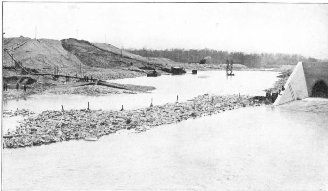
FIG. 214—BEGINNING HYDRAULIC FILL OF THE RIVER SECTION, ENGLEWOOD DAM, APRIL 5, 1920
