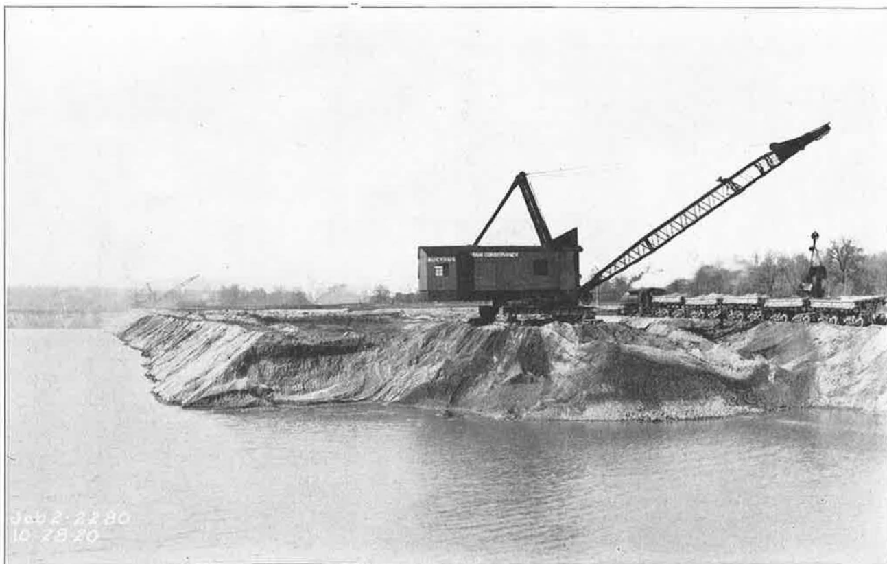
FIG. 273—DRAGLINE EXCAVATOR DIGGING MATERIAL IN ENGLEWOOD BORROW PIT, OCT. 28, 1920
