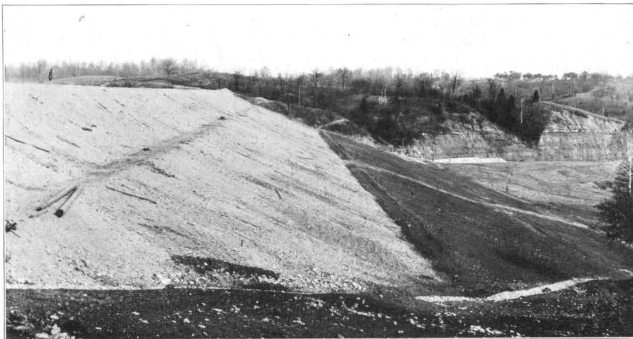
FIG. 245—THE DOWNSTREAM SLOPE OF THE GERMANTOWN DAM
