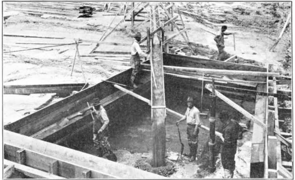
FIG. 32—FIRST CONCRETE AT ENGLEWOOD
