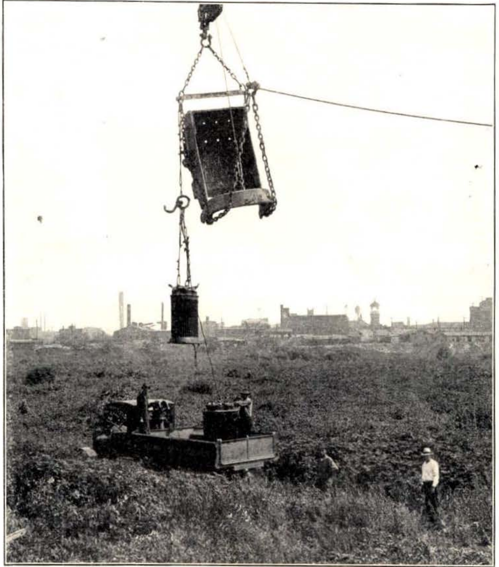
FIG. 41—A BIG DRAGLINE USED AS A DERRICK
