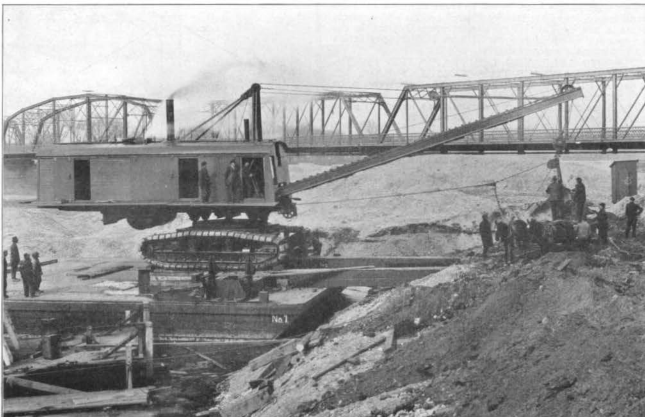
FIG. 127—CATERPILLAR DRAGLINE MOUNTED ON SCOW FOR MIAMI RIVER WORK, FEB. 27, 1919.
