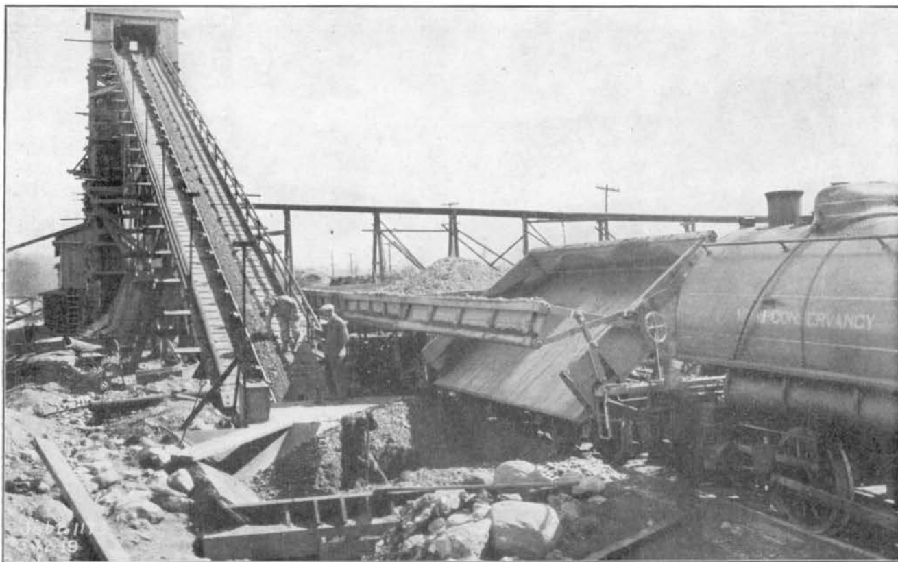
FIG. 115—STARTING THE GRAVEL THROUGH THE SCREENING AND WASHING PLANT.
