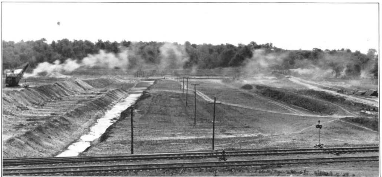
FIG 5—THE CUT-OFF TRENCH AT TAYLORSVILLE
