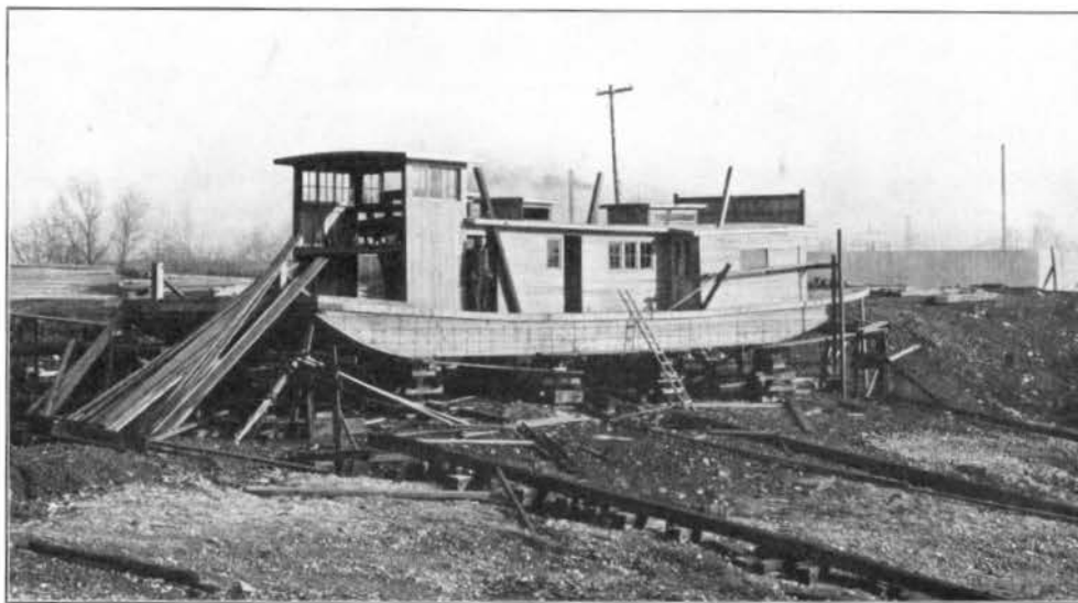
FIG. 98—STEAM TUG FOR LEVEE CONSTRUCTION, MIAMI RIVER
