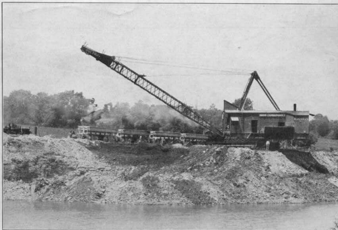
Excavating for Outlet Conduit at Englewood
