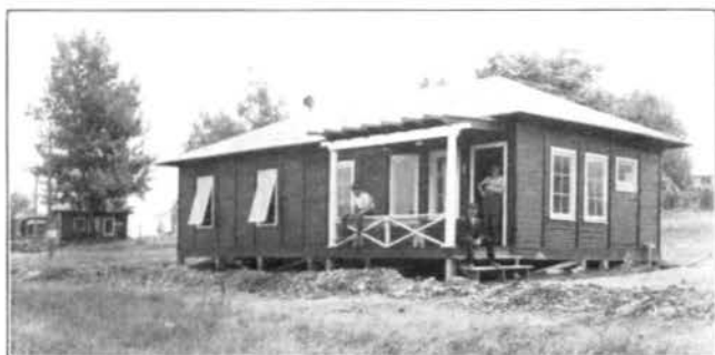
FIG. 14—A 12-MAN BUNKHOUSE AT HUFFMAN A one story house 18 by 42 feet in size, accommodating 12 men.
