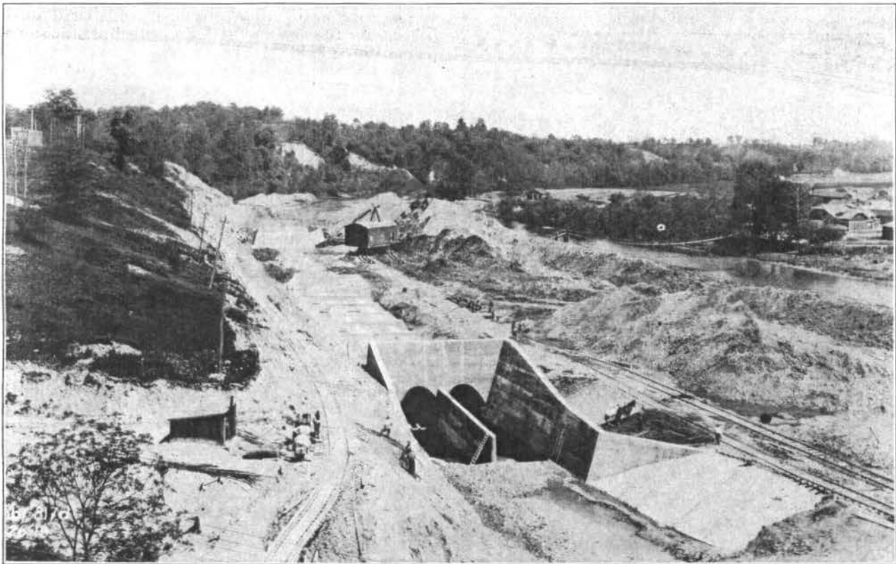
FIG. 158—ENTRANCE TO GERMANTOWN OUTLET CONDUITS, MAY 26, 1919.
