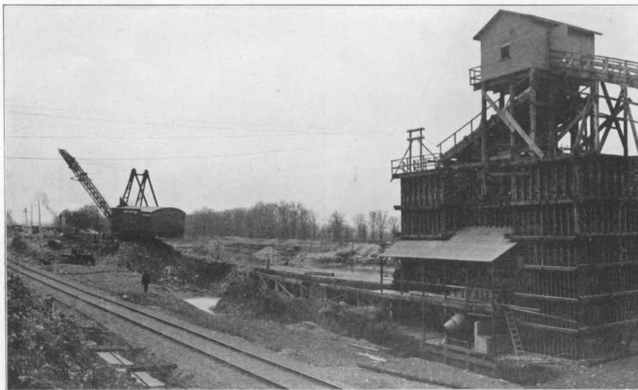
FIG. 69—EXCAVATION FOR CONCRETE STRUCTURE AT THE HUFFMAN DAM.
