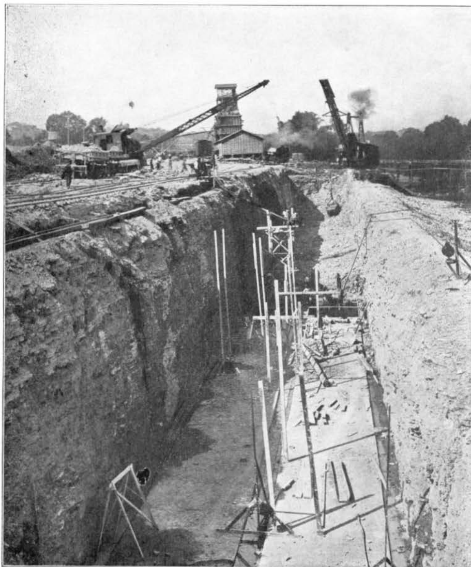
FIG. 57—EXCAVATION FOR THE CONDUITS AT ENGLEWOOD
