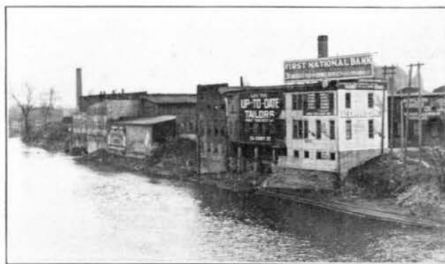
FIG. 23—BUILDINGS AT HAMILTON
