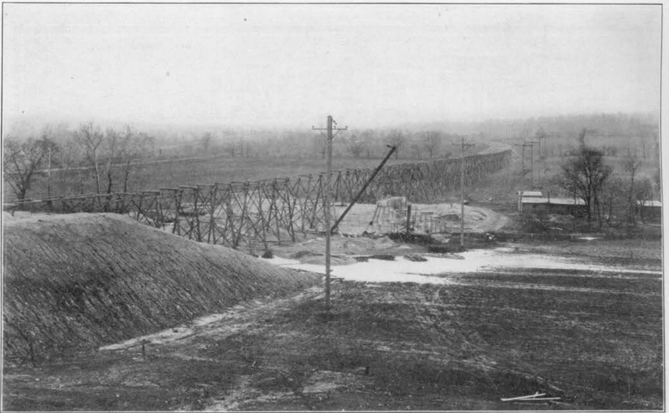
FIG. 88—CONSTRUCTION TRESTLE FOR THE FILL AT PICAYUNE CREEK, B. & O. R. R., JAN. 15, 1919
