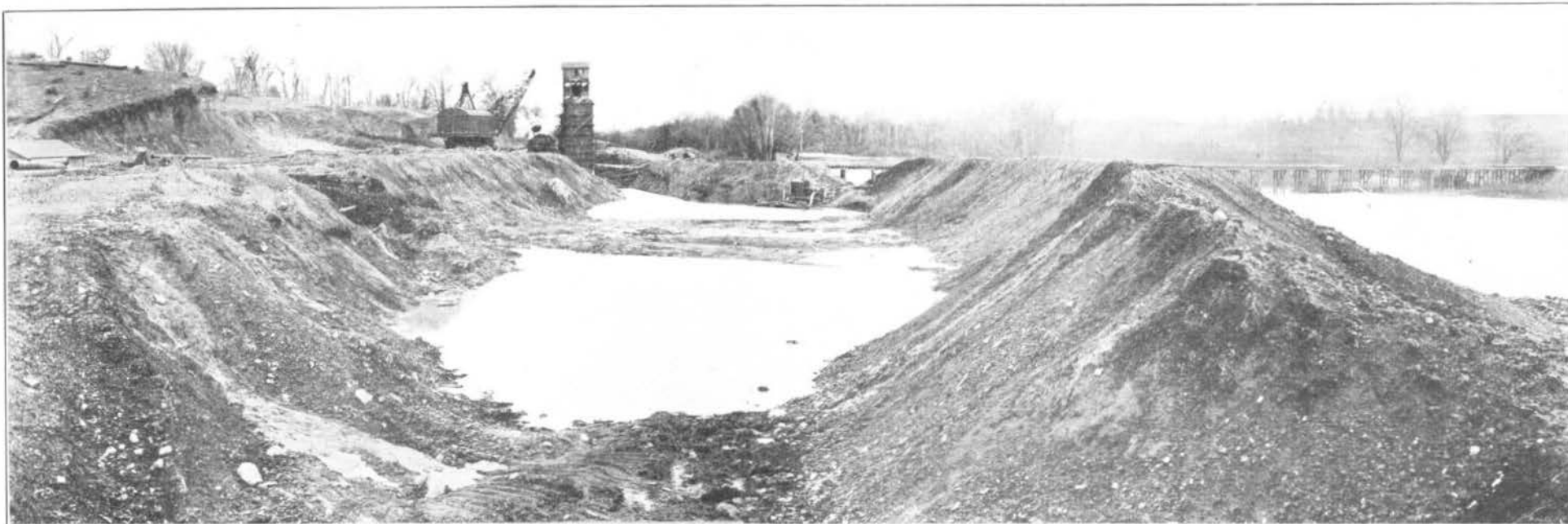
FIG. 73—COFFER DAM AND OUTLET CONDUIT EXCAVATION AT TAYLORSVILLE.
