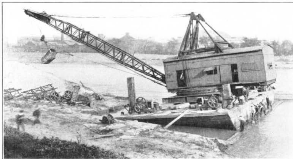
FIG. 151—DRAGLINE ON SCOW, DAYTON, MAY 14, 1919.
