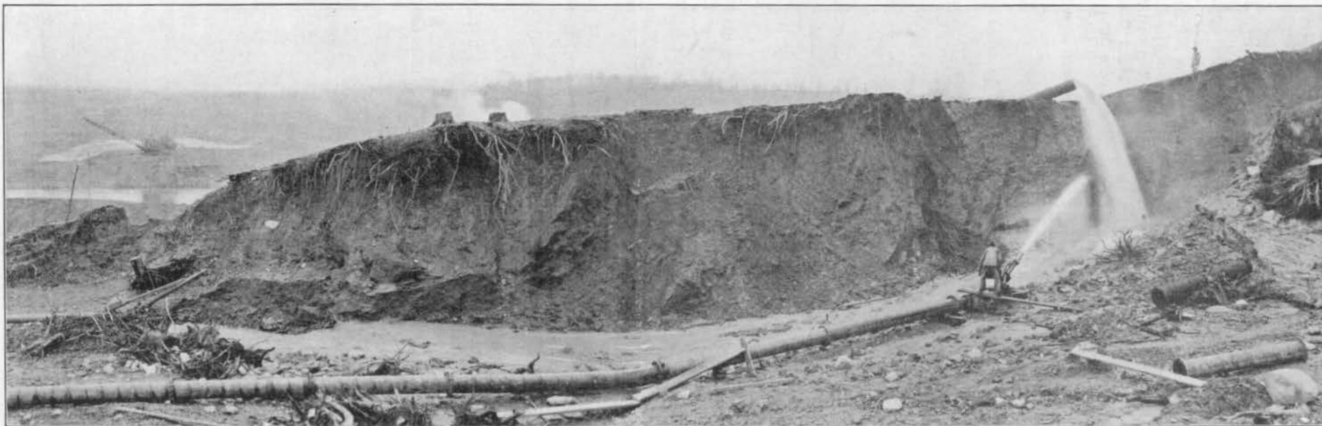
FIG. 86—THE HYDRAULIC FILL BORROW PIT, TAYLORSVILLE, DECEMBER 23, 1918.
