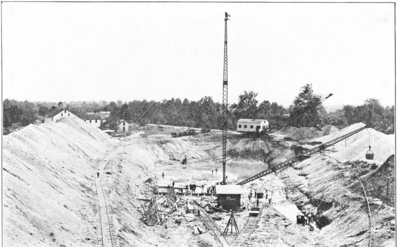
FIG. 30—EXCAVATION FOR ENTRANCE TO OUTLET CONDUIT AT LOCKINGTON
