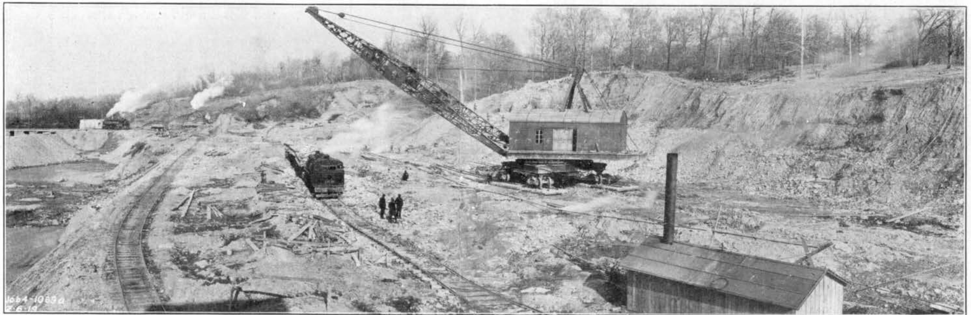
FIG. 112—EXCAVATION FOR OUTLET WORKS, TAYLORSVILLE, FEBRUARY 6, 1919.
