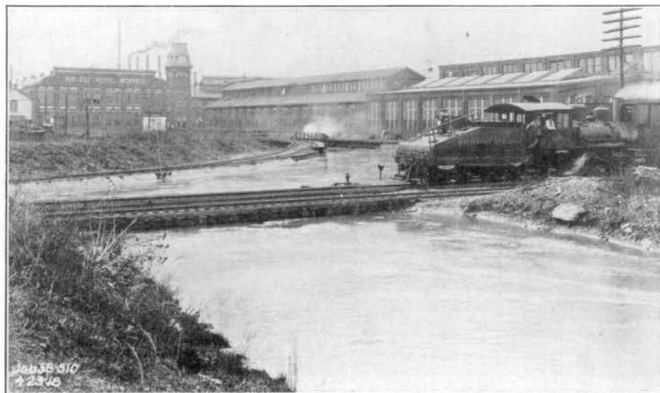
FIG. 96—B. & O. CROSSING, HYDRAULIC CANAL, HAMILTON, APR. 23, 1918.
