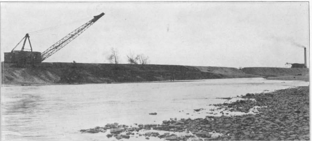
FIG. 63.—THE NEW MIAMI RIVER LEVEE AT HAMILTON
