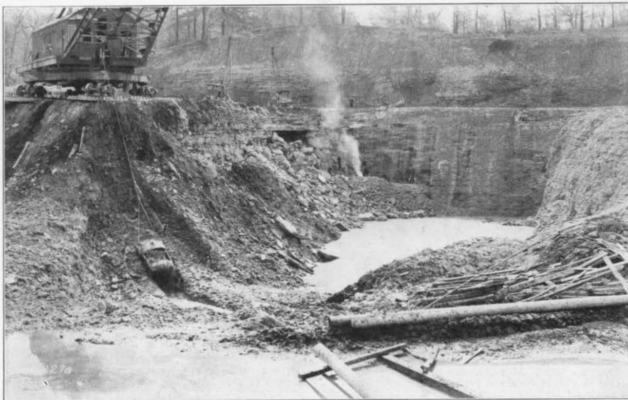
EXCAVATING FOR THE HYDRAULIC JUMP POOL AT TAYLORSVILLE, MAY 13, 1919.
