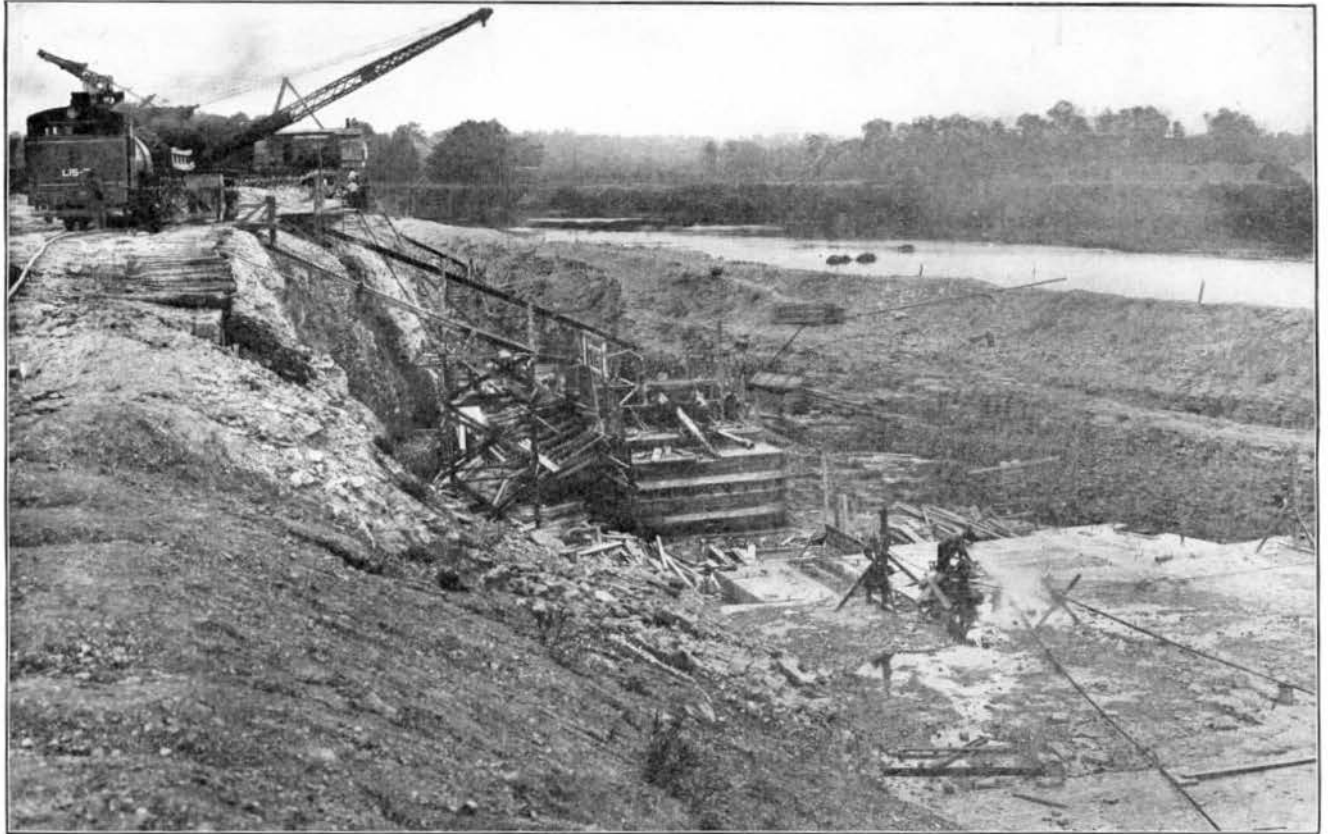
FIG. 34—CONCRETING OUTLET CONDUITS AT ENGLEWOOD—VIEW LOOKING UP STREAM
