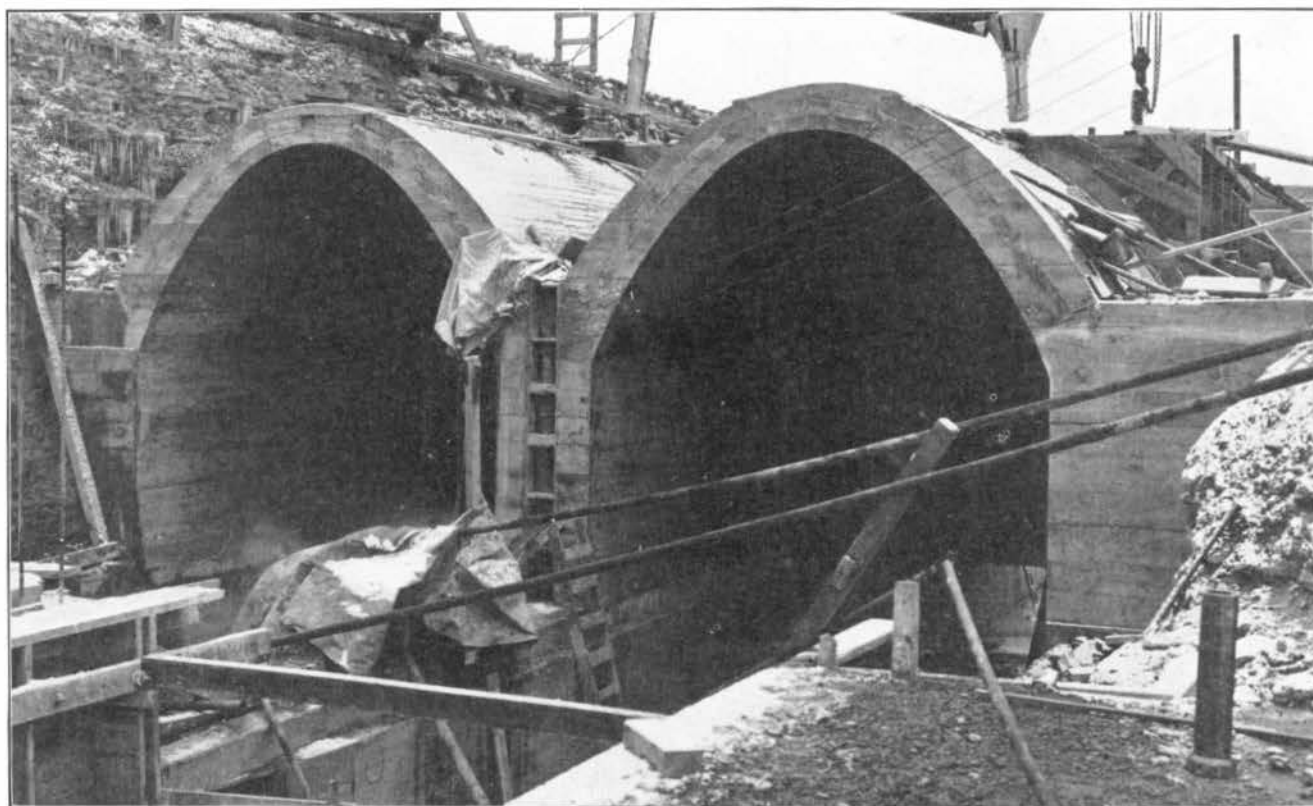
FIG. 82—FINISHED SECTION OF CONDUITS, ENGLEWOOD, DECEMBER 26, 1918.
