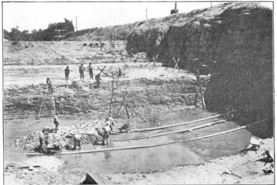
FIG. 33—EXCAVATION FOR POOL CHAMBER AT ENGLEWOOD
