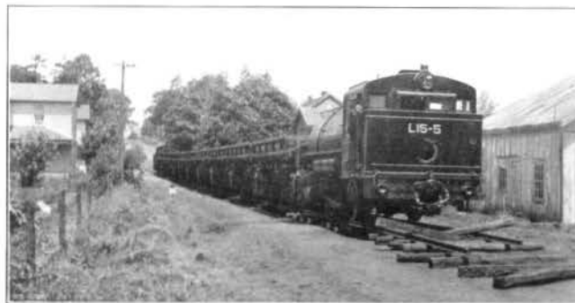
FIG. 16—MOVING A CONSTRUCTION TRAIN TO GERMANTOWN DAMSITE
