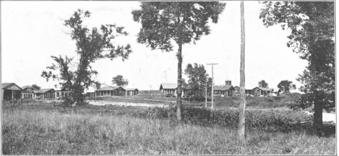
FIG. 77.—THE COMPLETED CAMP AT LOCKINGTON
