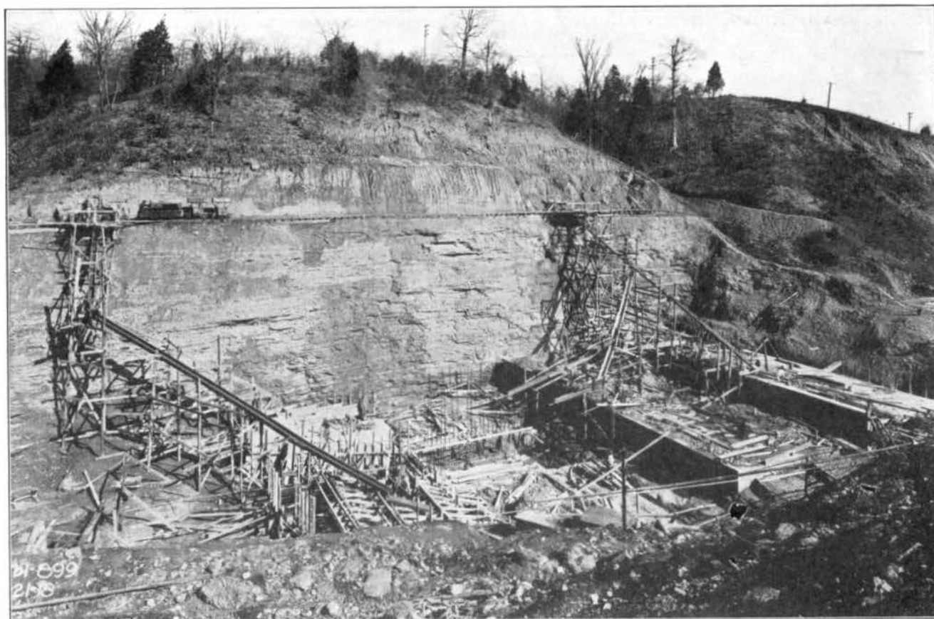
FIG. 60—CONCRETING THE OUTLET STRUCTURE AT GERMANTOWN
