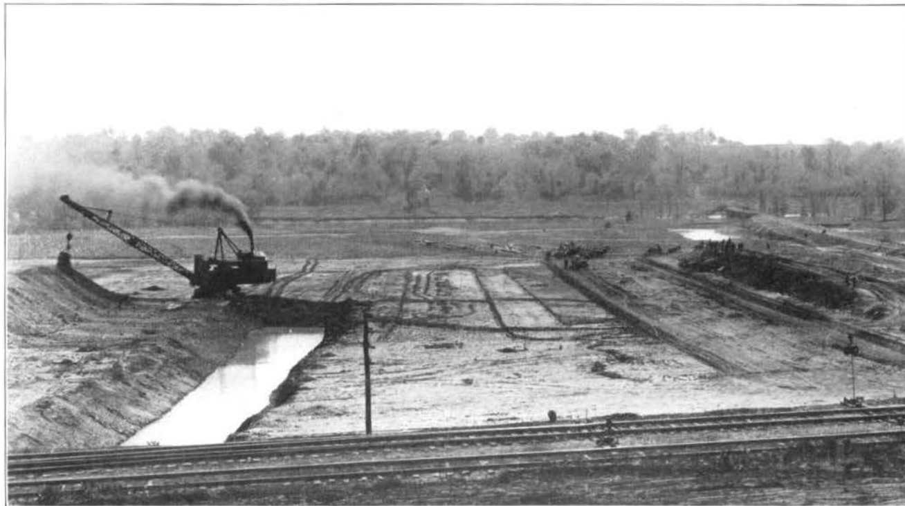
FIG. 6—EXCAVATING CUT-OFF TRENCH AT TAYLORSVILLE
