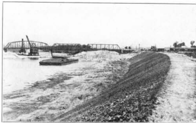
FIG. 25—NEW LEVEE AT DAYTON
