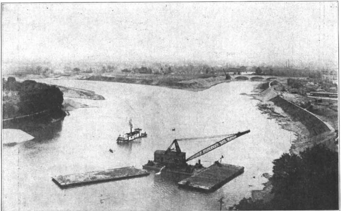
THE MIAMI RIVER AND THE NEW LEVEES
