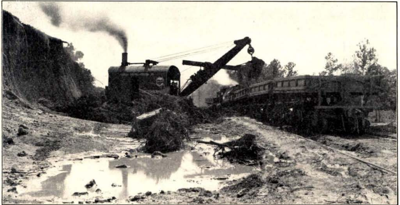
FIG 44—MARION MODEL 36 STEAM SHOVEL EXCAVATING THE EAST BANK OF THE MIAMI AT TAYLORSVILLE
