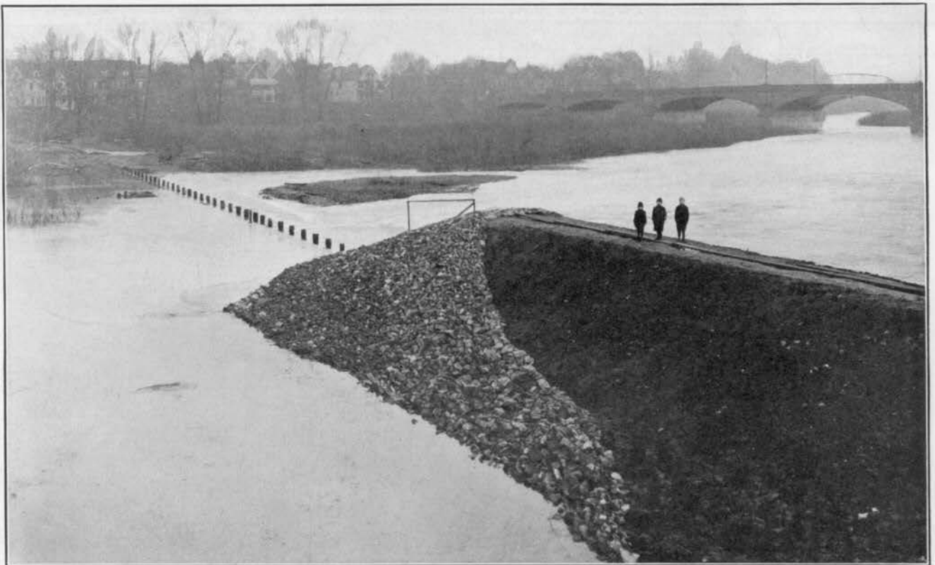
FIG. 89—SUNSET AVENUE DAM, DAYTON, DEC. 11, 1918.
