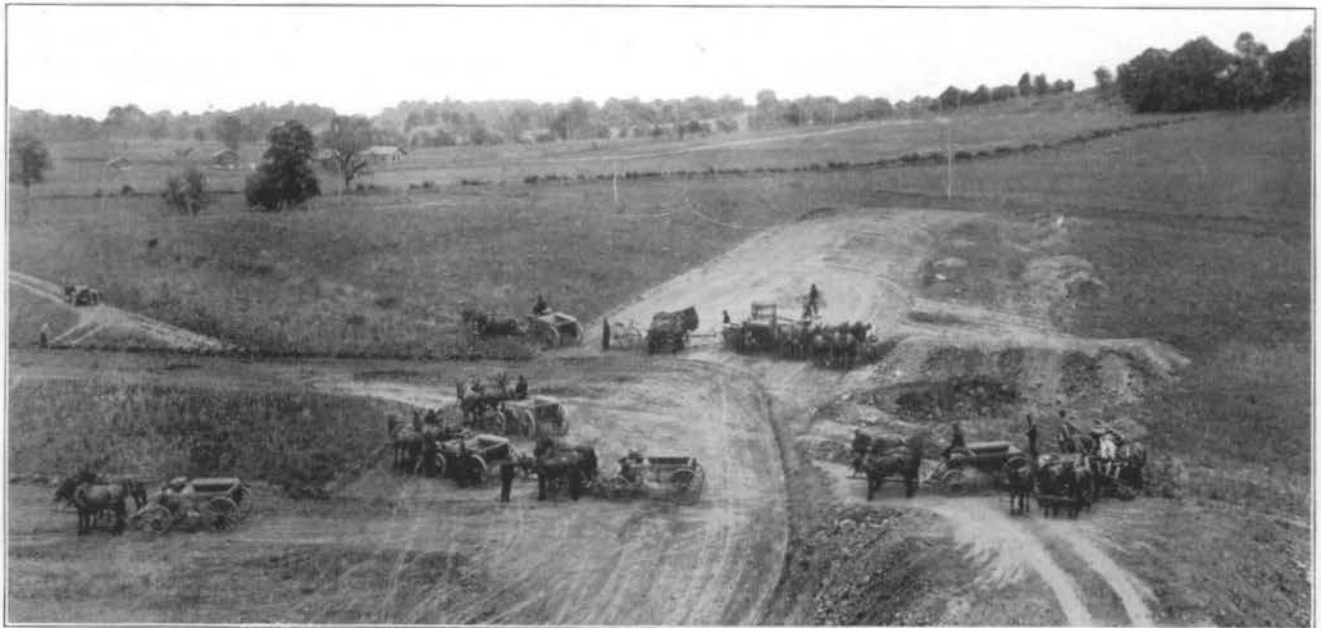
FIG. 2—STRIPPING THE DAMSITE AT ENGLEWOOD
