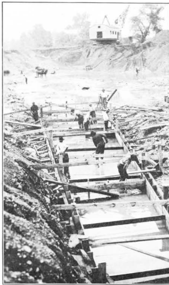
FIG. 31—FIRST CONCRETE AT LOCKINGTON
