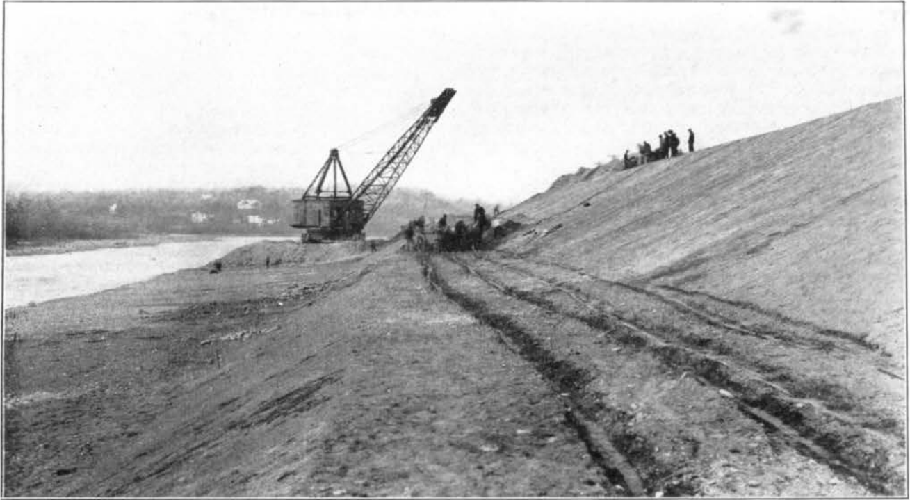
FIG. 109—FINISHING THE LEVEE AT HAMILTON, FEB. 7, 1919.
