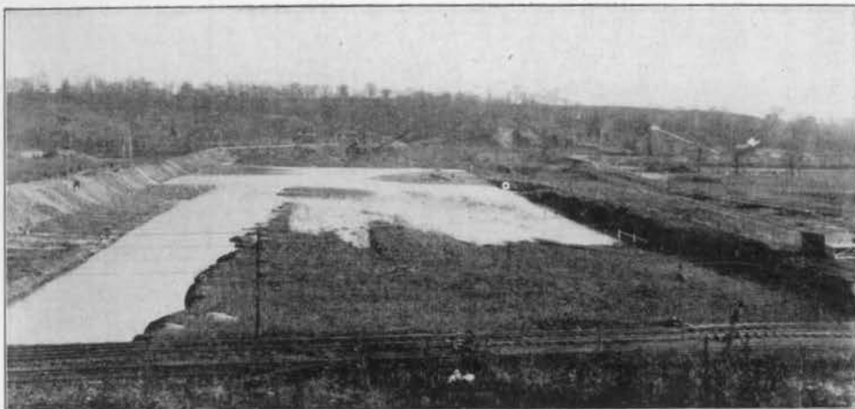
FIG. 84—HYDRAULIC FILL POOL, TAYLORSVILLE, DECEMBER 16, 1918.
