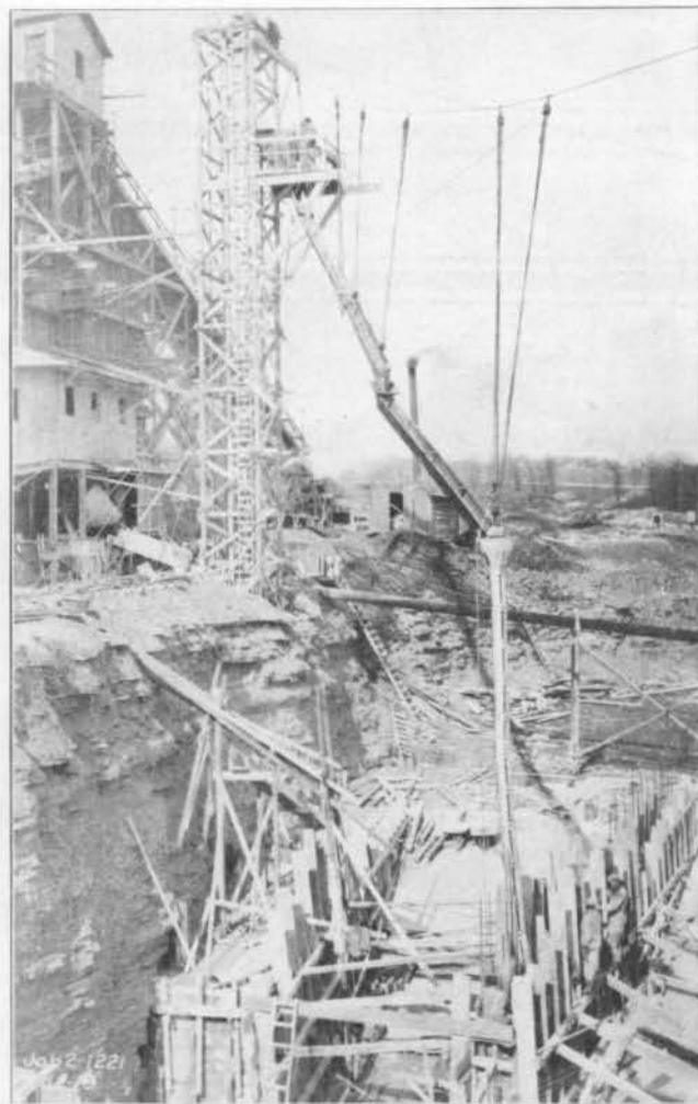
FIG. 145—CONCRETING TOWER, ENGLEWOOD
