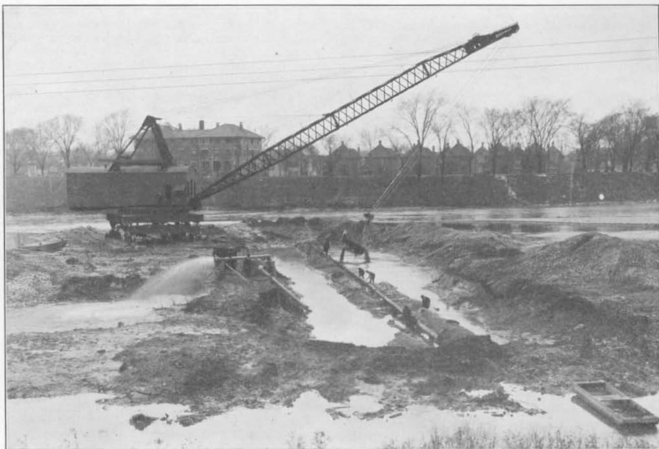
FIG. 70—LOWERING A 12" WATER PIPE IN THE MIAMI RIVER AT DAYTON.
