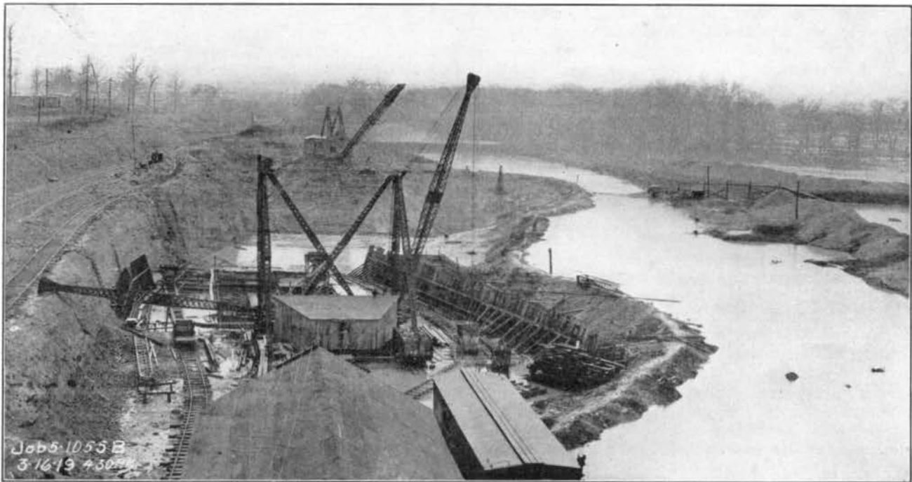
FIG. 116—THE WORK AT HUFFMAN DURING THE FLOOD, MARCH 16, 1919.
