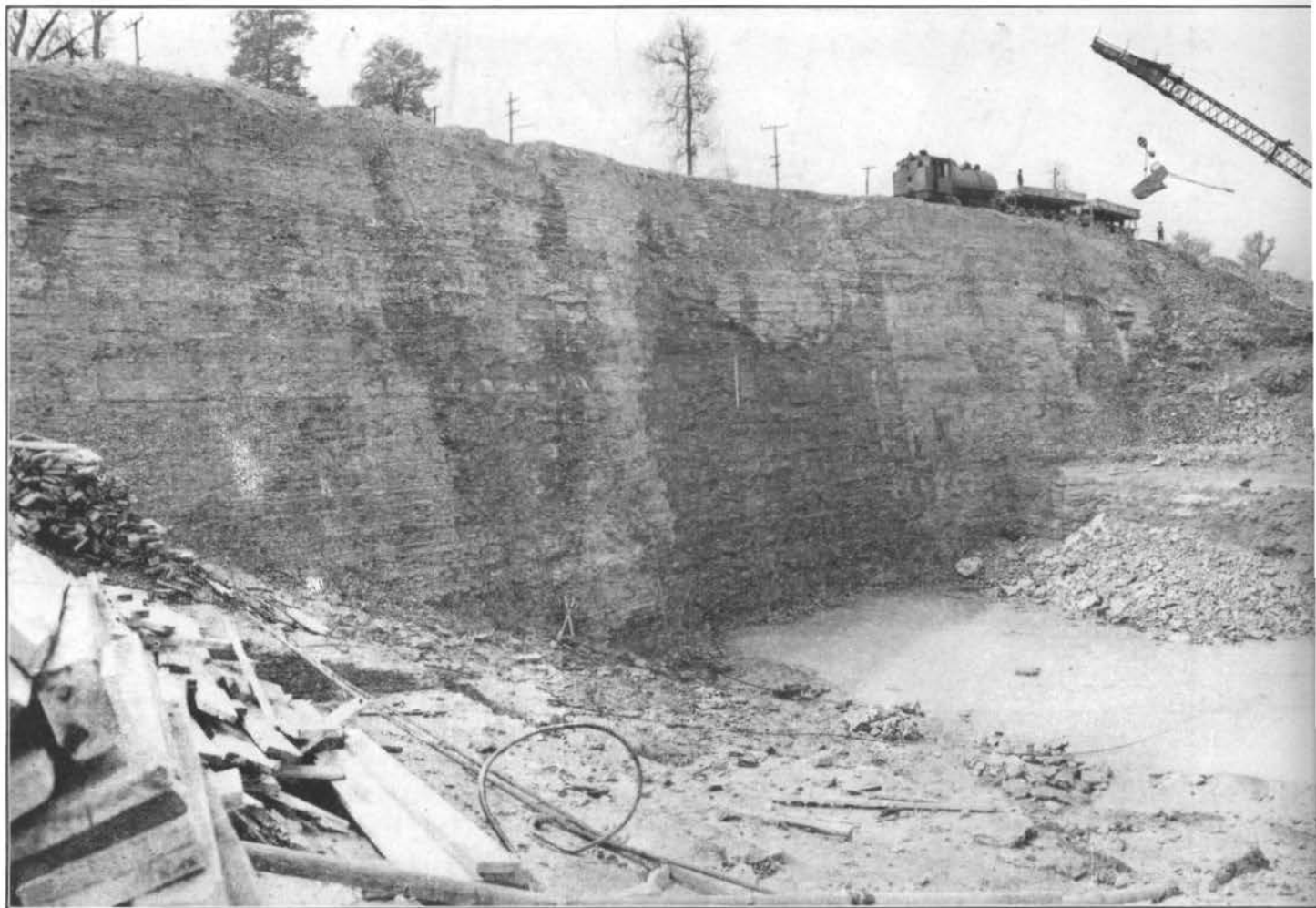
FIG. 149—EXCAVATION FOR OUTLET WORKS BELOW CONDUITS AT THE HUFFMAN DAM, MAY 1
