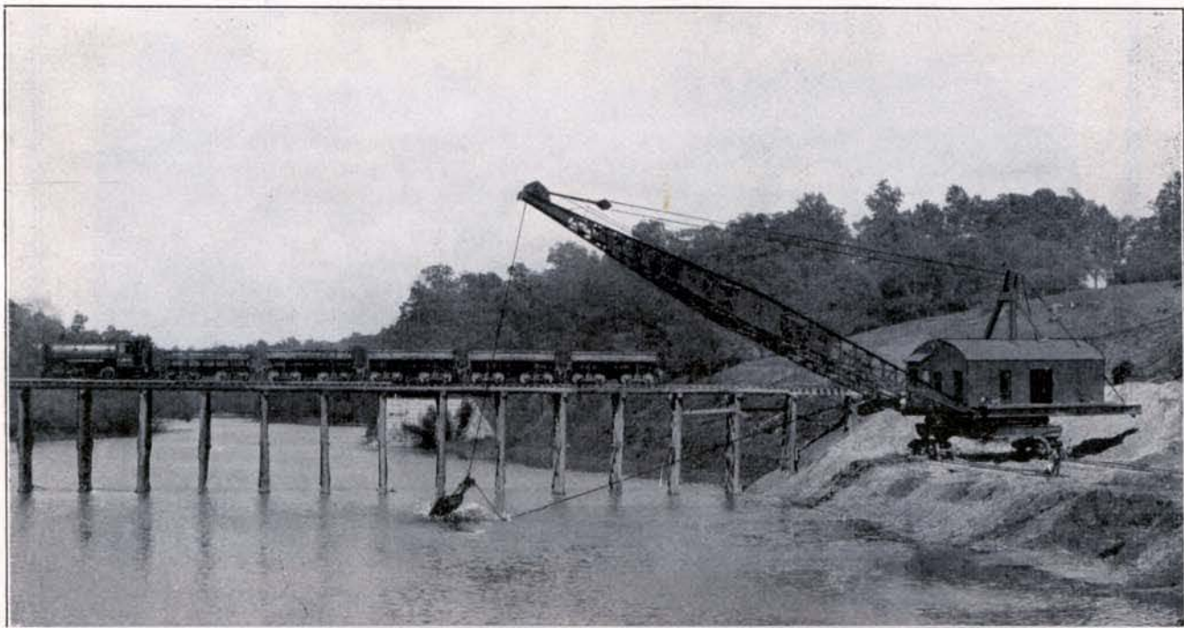
FIG. 39—LIDGERWOOD DRAGLINE EXCAVATING CUT-OFF TRENCH IN THE MIAMI RIVER
