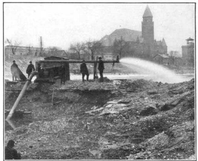
FIG. 99—PORTABLE PUMPING OUTFIT USED ON CONSERVANCY WORK
