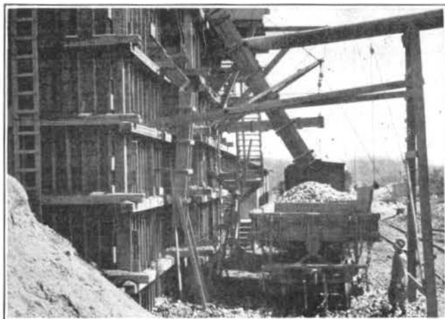
FIG. 124—DISCARDING THE UNFIT MATERIALS AT THE ENGLEWOOD SCREENING AND WASHING PLANT.
