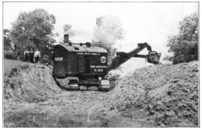
FIG. 3—RAILWAY EXCAVATION AT GER-MANTOWN
