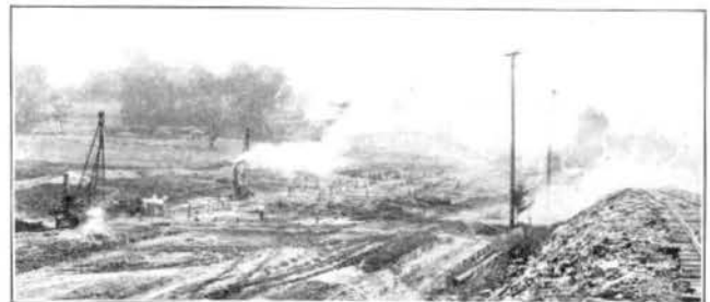
FIG. 28—DRILLING BLAST HOLES AT HUFFMAN
