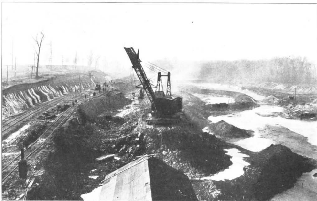
EXCAVATING FOR OUTLET CHANNEL, HUFFMAN DAM, JAN. 16, 1919. SEE PAGE 108.
