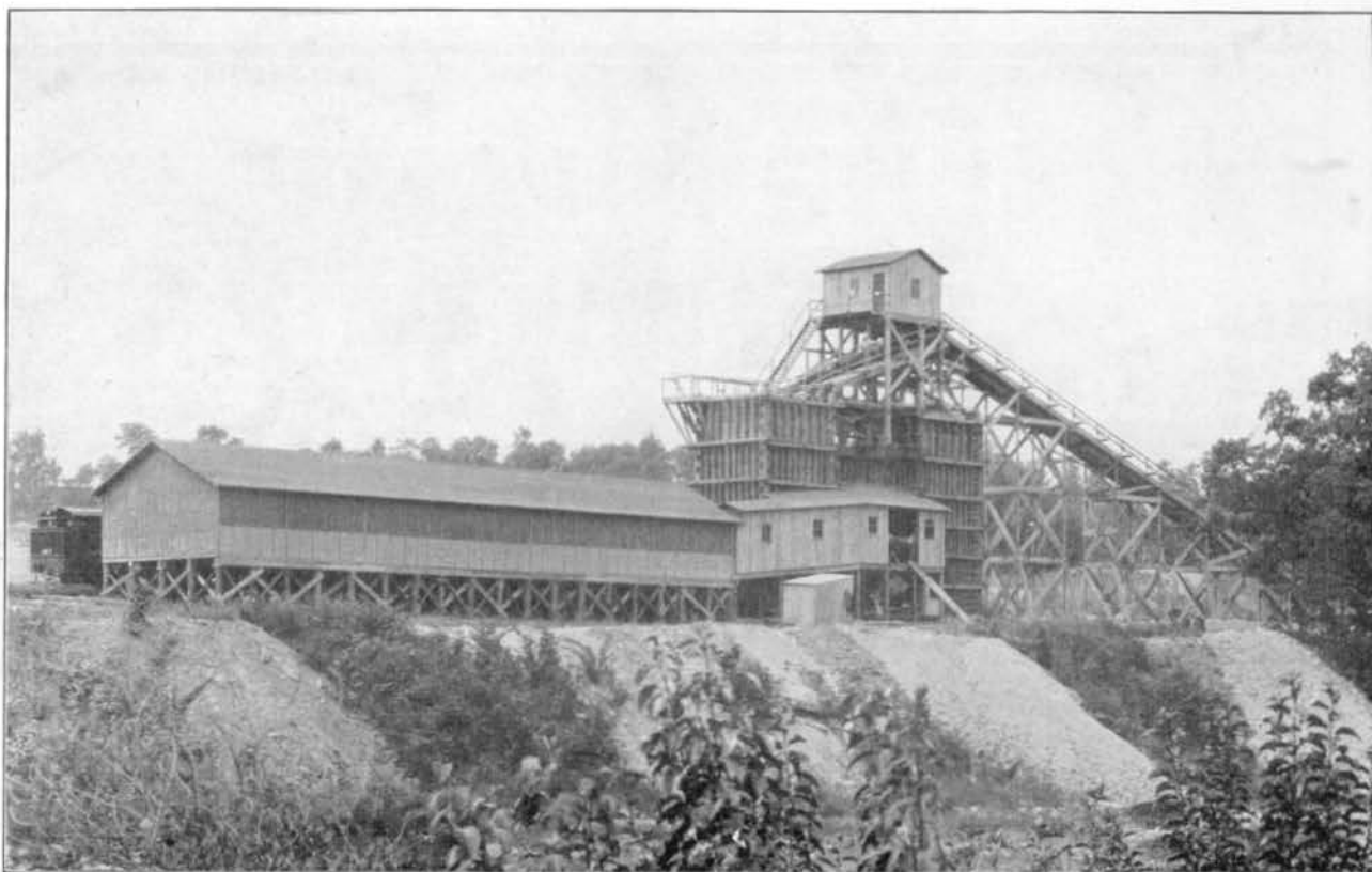
FIG. 114—GRAVEL WASHING AND SCREENING PLANT AND CEMENT HOUSE, ENGLEWOOD, JULY 15, 1918.
