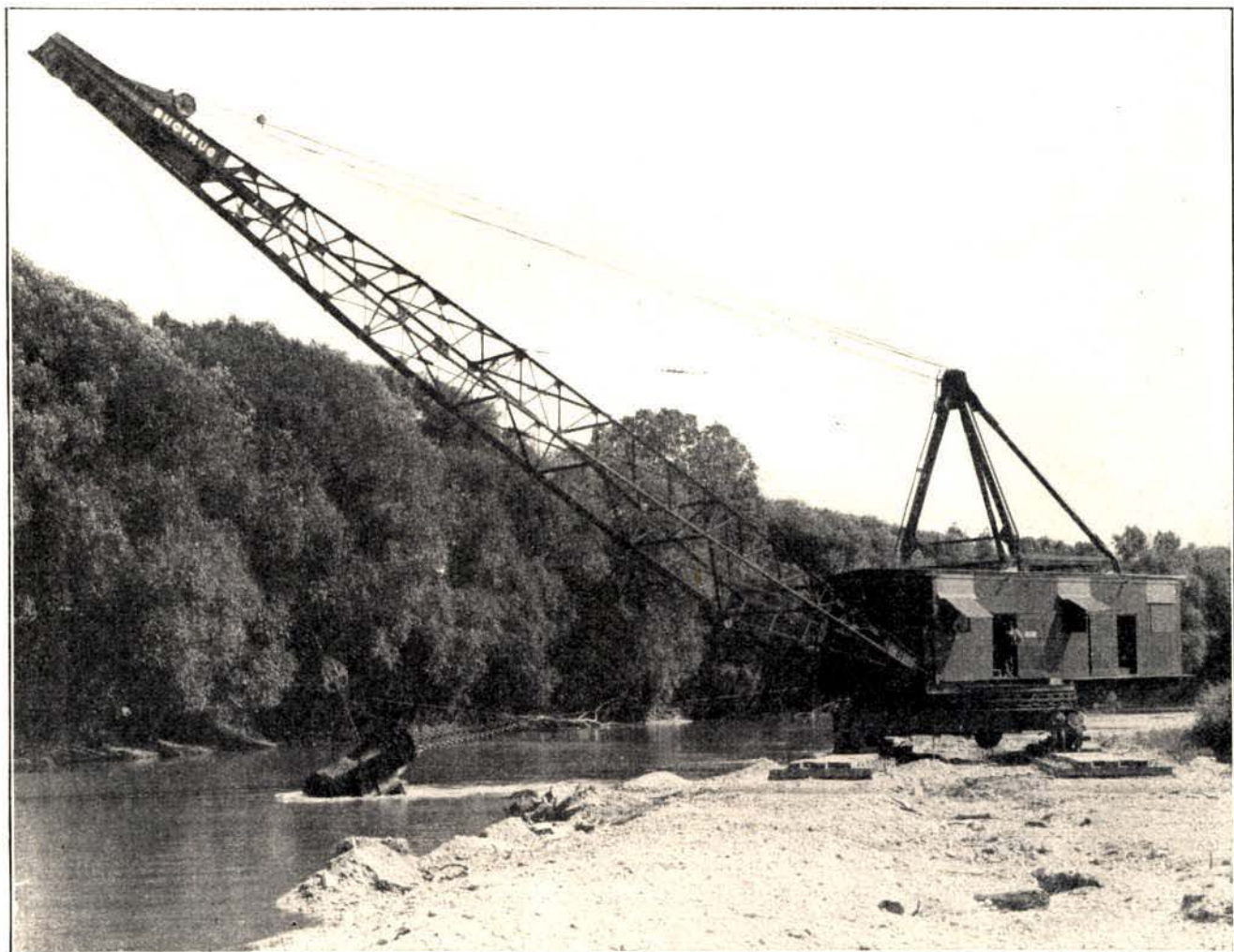
FIG 43—DRAGLINE BUCKET COMING UP FROM BOTTOM OF THE MIAMI RIVER WITH A LOAD
