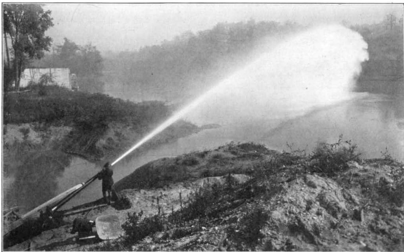
FIG. 59—TESTING THE HIGH PRESSURE PUMPS FOR THE HYDRAULIC FILL AT TAYLORSVILLE The same "giant" (at the left) which will tear down the earth to make the fill. (See page 57.)
