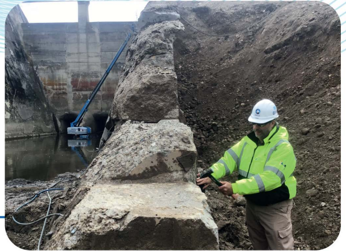
Inspecting concrete during rehab work on Lockington Dam.
