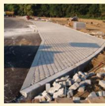
Pervious brick pavers are installed to allow runoff to seep into the ground.
