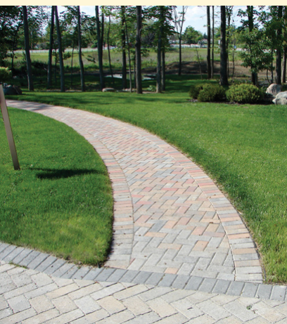
Above: Pervious paver bricks are used for the driveway as well as the driveway apron and pedestrian sidewalks.
